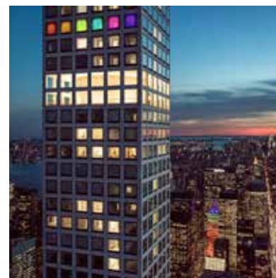
Photos courtesy of Durston Saylor
